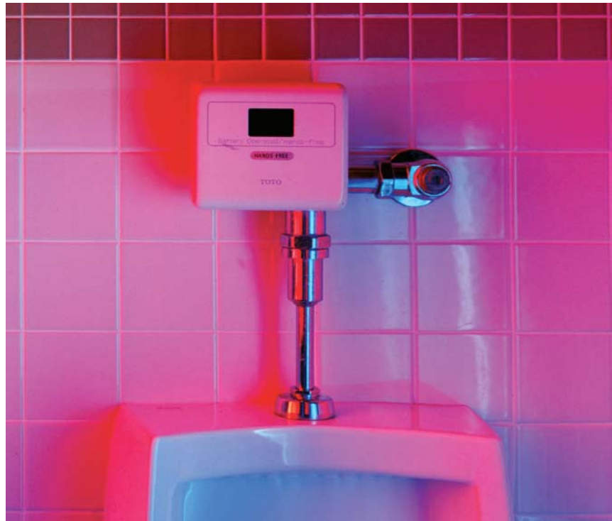
Fig. 1: Installation of the automatic flush system
